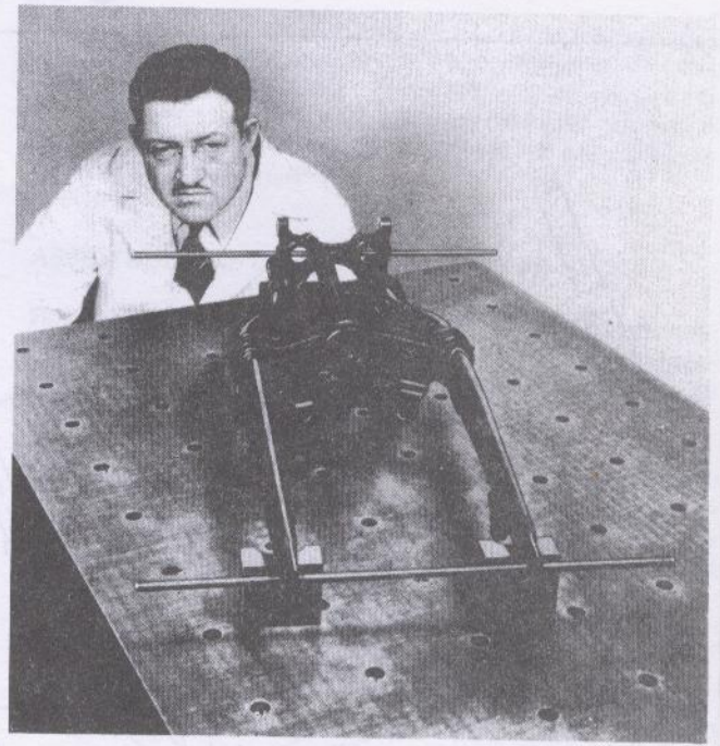
ILLUS. 58 (ABOVE)—CORRECT ALIGNMENT OF FORK SIDES WITH FORK STEM.
